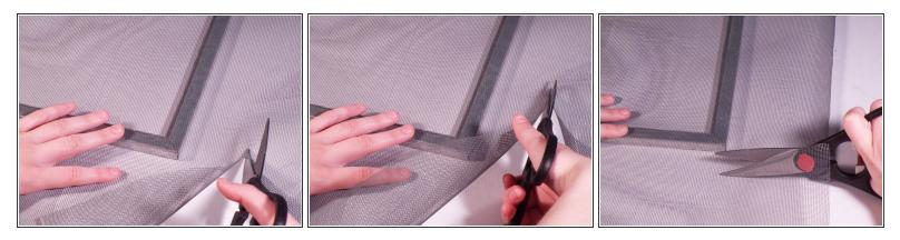
Use a pair of scissors or a utility knife to cut off from the roll of mesh, leaving around an extra inch outward from the frame.
