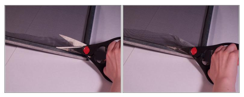
• Cut off the excess mesh with the pair of scissors or utility knife.
