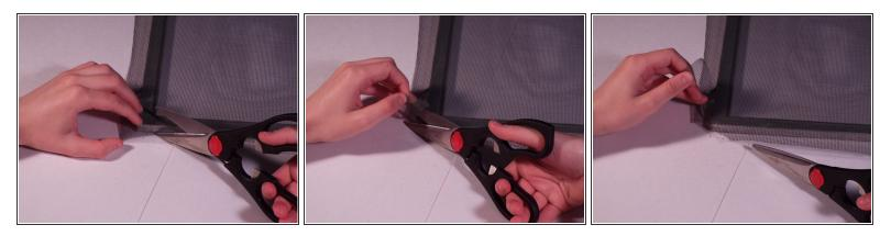
• Cut off the corners of the mesh diagonally and leave a bit of extra mesh over the frame.
