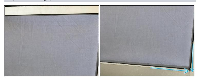
Check the pool cage for any problems with the newly attached screen. The new thread should be pressed firmly into the pool cage, and the screen should be pulled tight so there are no wrinkles.
