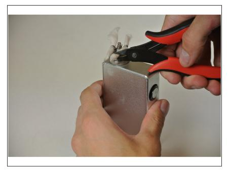
Using the wire cutters, cut cotton approximately ¼ of an inch away from outside of atomizer on each strand.
