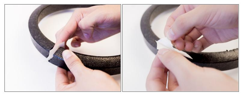
• Peel off double sided tape and apply to one side of the broken hull.
