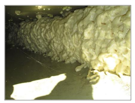
The amount of foam pictured was the contents of two cans. Don't worry if small gaps remain as the unexpanded foam "plops" into the cavity. As it expands, the foam will fill in and "rise" on the open side.
