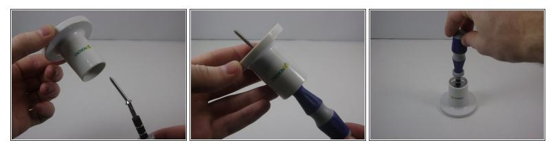
• Place the screw through the bracket, as shown, and screw it into the marked or drilled location.
