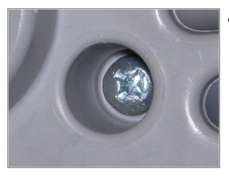
With a Phillips head screwdriver, remove all (4) of the screws.
