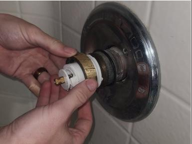
Remove the metal ring using a pair of channel lock pliers and twisting counter clockwise.
