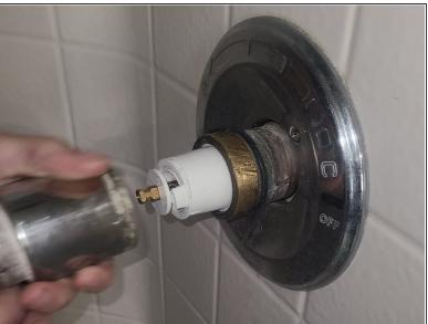
Remove the metal sleeve by grasping with one hand and pulling towards your body.
