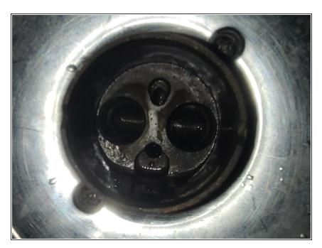
Do one last double check for any objects that will interfere with the installation of the new cartridge.
