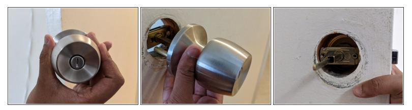
• Grab the exterior knob and align it with the holes of the latch and push it in from the side of the door that is outside your room.
