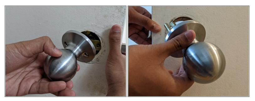
• Once the screws are off, safely pull out the doorknob from both sides.
