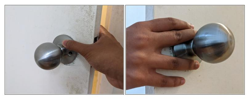
A Hold both sides of the current doorknob with a hand to prevent it from falling out in the removal process.
