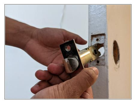
• Pull the latch out of the hole it is secured in.
