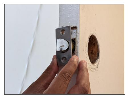
Insert the new latch into the designated latch hole after figuring out the correct way to face it.
