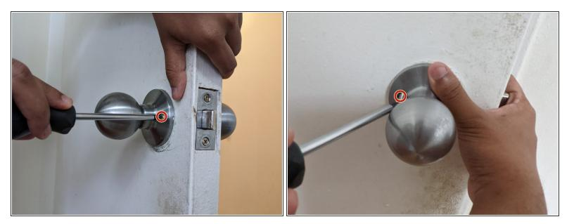
Using a Phillips #2 screwdriver, remove the two screws from the passage doorknob.
