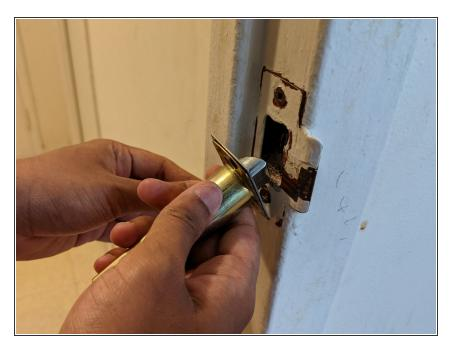
• Grab the new latch that comes with the privacy doorknob set and ensure the flat side is facing away from the closing direction of the door.
