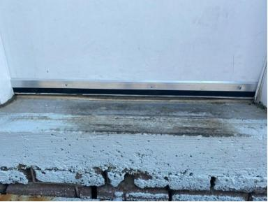
• Install the Door Sweep by drilling it in using a cordless drill.
