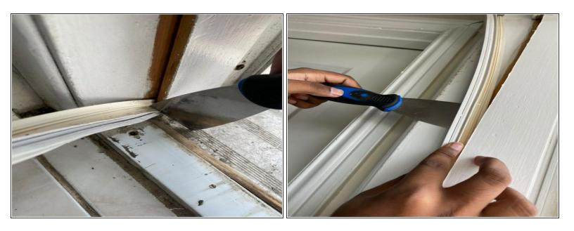
Using the putty knife, push the new weatherstripping into the door groove.
