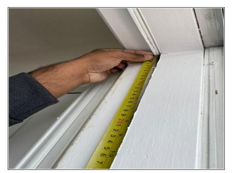
After removing the weatherstripping, measure the door frame using the measuring tape.
