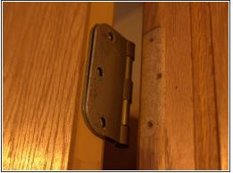
Using the Phillips #2 screwdriver, remove the screws from the doorframe. Repeat steps 2 and 3 for all of the hinges.
