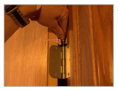
Pull out the pin out of the hinge.
