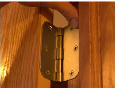
With the new door, screw in the new hinges in the doorframe in the same place the old ones were.
