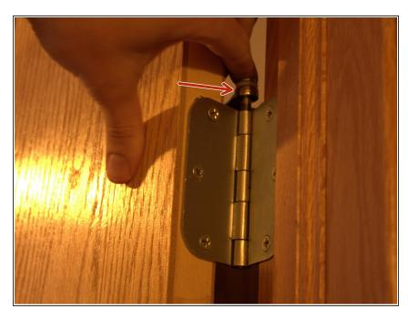
Push the pin back into the hinge to make its secure. Repeat steps 4 and 5 for all the hinges.
