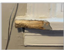
Remove any loose, splintered, or jagged wood by hand.
