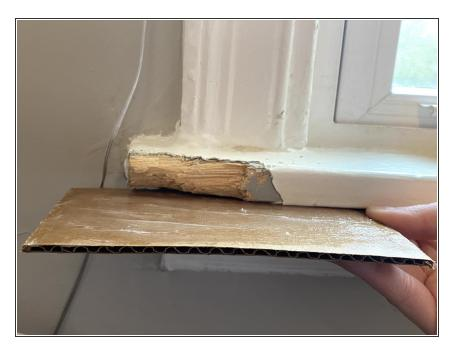
Hold one section of cardboard underneath the corner needing repair with the Vaseline side facing up.
