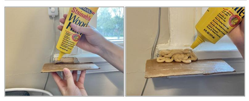
Apply wood filler to the corner by squeezing the tube.
