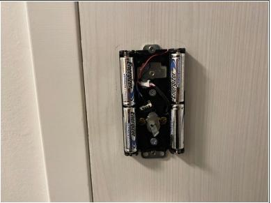
Install four AA batteries in the battery pack.
