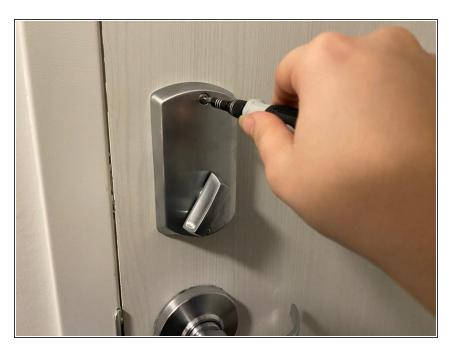
Use the Phillips #1 screwdriver to tighten the screws.
