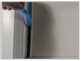
With the non-beveled putty knife (or your fingernail) lift up and remove the blue covering from the glazing tape on all 4 sides.
