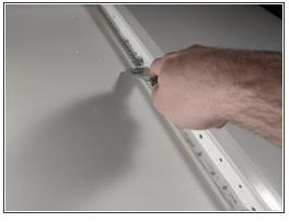
Using the beveled putty knife, scrape away most of the leftover glazing tape from the frame.
