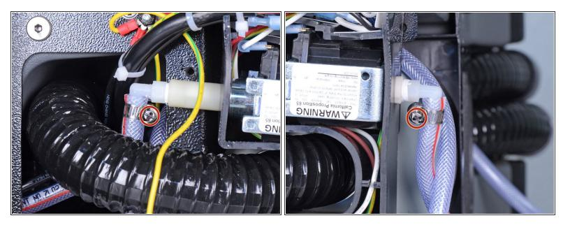
Use a flathead screwdriver to loosen the hose clamps at both ends of the pump.
