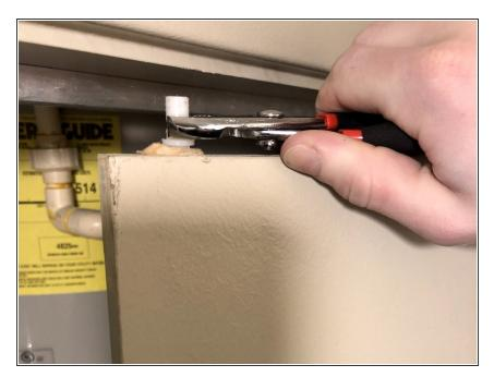
Remove the current pin with pliers.
