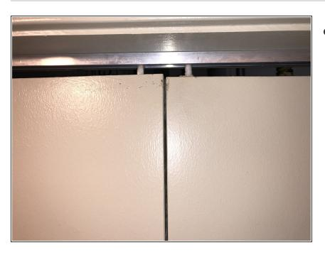
When completed, the bifold doors should close and be positioned within the tracking.
