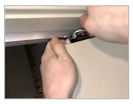
Secure the pin within the tracking using the pliers.
